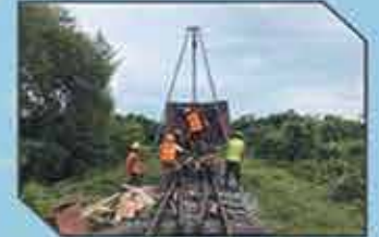
Karoppi Bridge Railway Project
